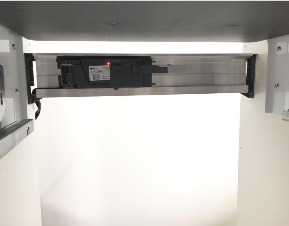
Blum Servo Drive installed behind Concelo Bin Unit.
